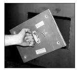
4. Insert the door into the opening at an angle and then center the door.
