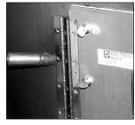
7. Install the fasteners with washers. For hinged door, position hinge on duct wall and plug weld.
